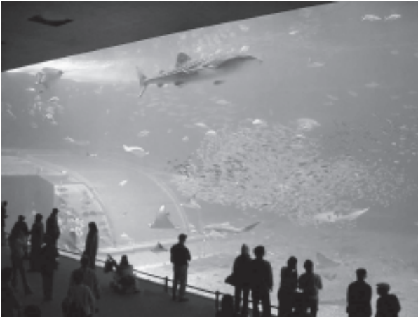
Figure 5.5. The Whale Shark exhibit (7,500 m 3 total volume) incorporating the world's largest acrylic window (22.5 m long x 8.2 m high x 0.6 m thick): Okinawa Expo Aquarium, Japan.
