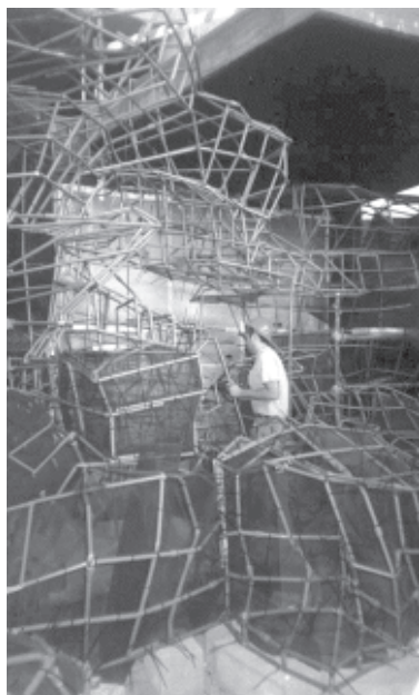
Figure 5.8. Construction of artificial rockwork armature using PVC piping, prior to attachment of plastic mesh: Oceanário de Lisboa, Lisbon, Portugal (Photograph courtesy of the David L. Manwarren Corp.).
